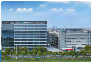
Suzhou R&D and Production Base
